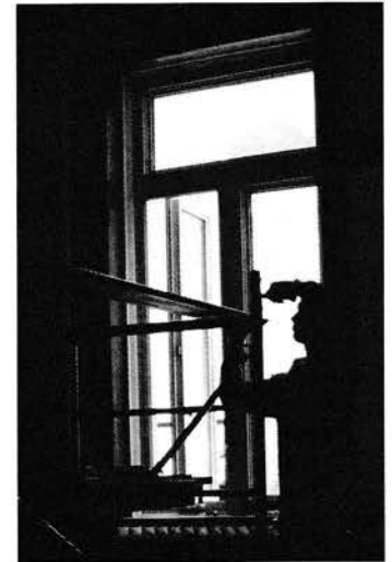
Work continues on the Fr. Freeland room.
